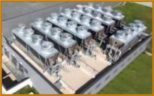
Seven dry-hybrid cooling towers
