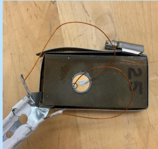
Installed LWR technology--monitoring
